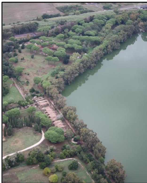
Aerial view over the northern sides of the hexagonal basin at Portus, showing the position of the Palazzo Imperiale (upper left) and the shipyard building (beneath the trees at the top of the photo).
