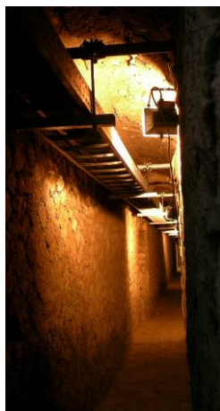
The Roman primary drainage network has been reinstated in order to collect and drain water
